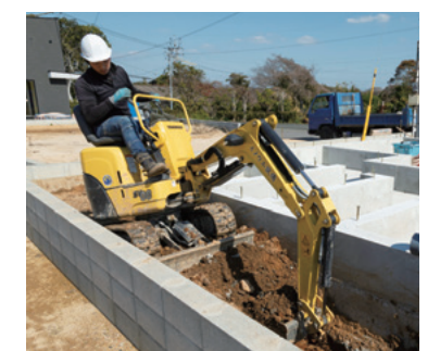
Efficient work even in narrow spaces
