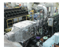
SCR system installation on test bench
