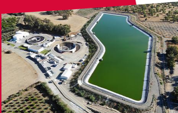
Guzelyurt Waste Water Treatment Plant, TURKEY
