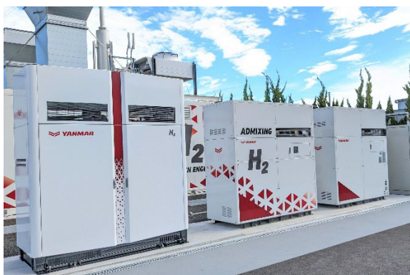
Left: From left to right, Hydrogen Fuel Cell Power Generation System, Hydrogen Mixed combustion CHP, and gas CHP; Right: 2G Hydrogen Fuel Engine CHP
