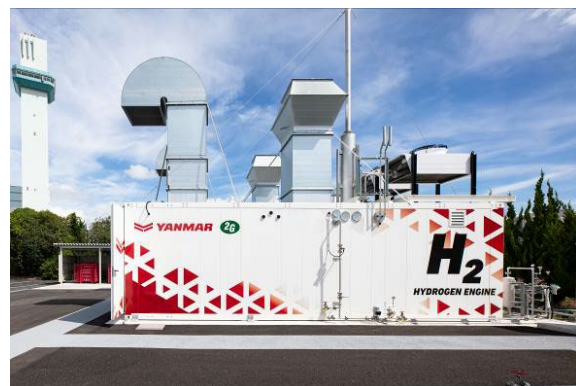
Left: From left to right, Hydrogen Fuel Cell Power Generation System, Hydrogen Mixed combustion CHP, and gas CHP; Right: 2G Hydrogen Fuel Engine CHP
