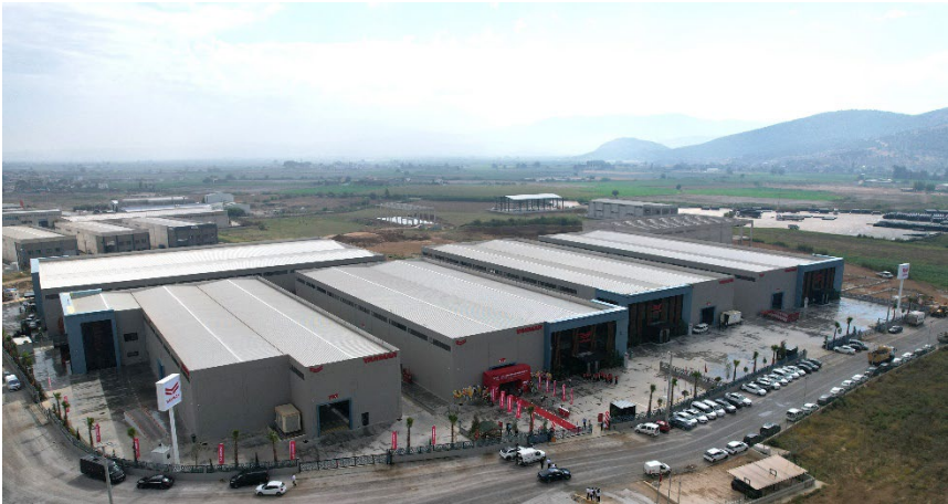
The new Yanmar Turkey manufacturing plant located in Izmir, Turkey.
